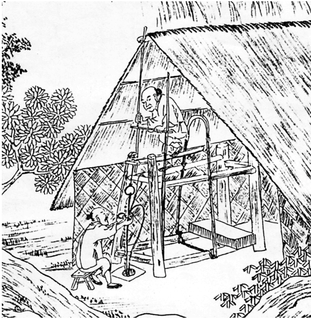
Ill. 17: Drilling a brine well at the Nanlang saline, Sichuan, early twentieth century
